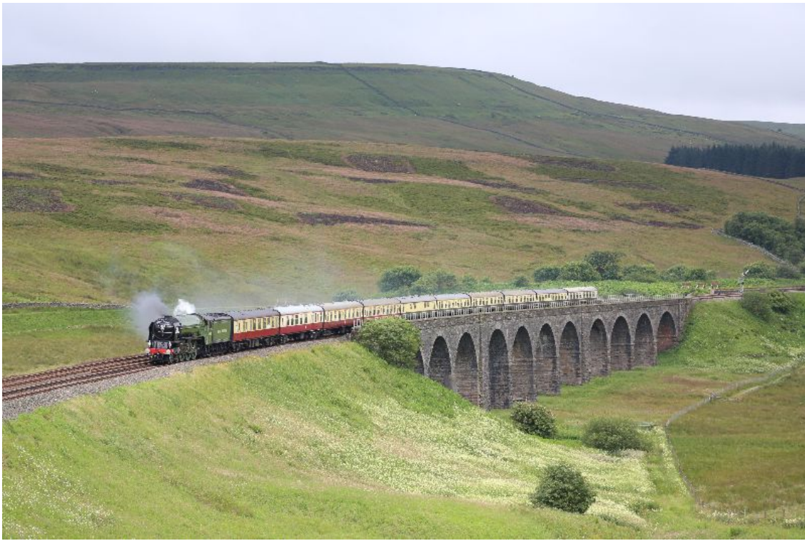
July 2019 - Tornado hauling 'The North Briton' across the Dandry Mire viaduct - Neil Wroe/A1SLT
