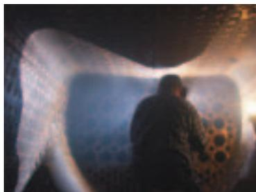
...and are welded to the firebox tube plate
