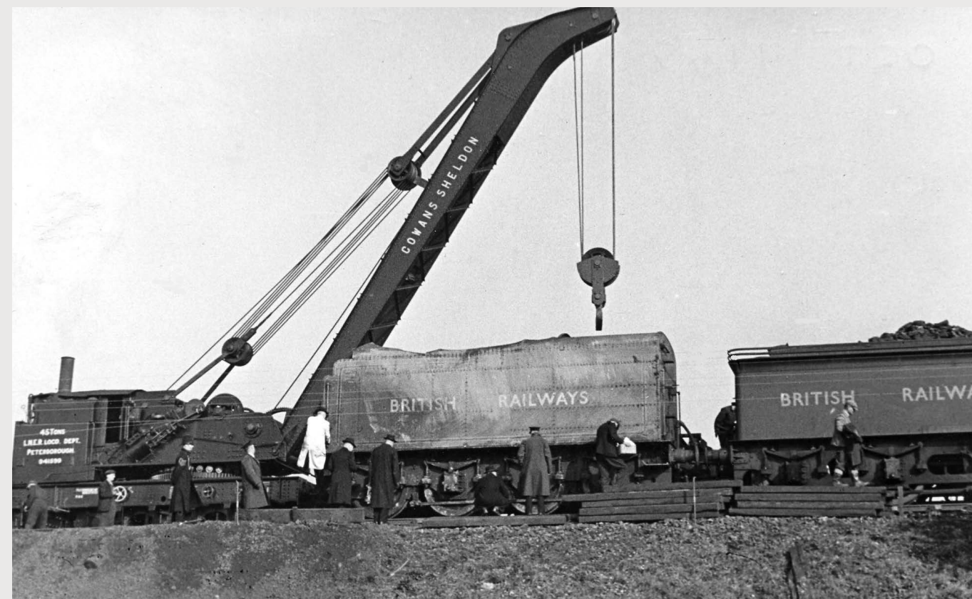
No. 60123's tender after being righted by the Peterborough Loco Dept. breakdown crane.
