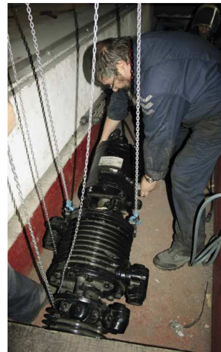
Rear air pump is lowered into pit.
