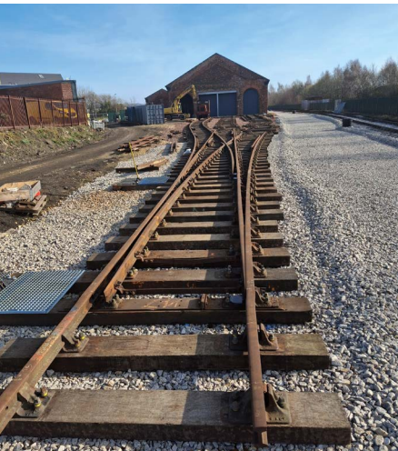
Above: Pit boards have been installed at the outside pit allowing rail traffic to run over them and allows us to maintain the pit. It also gives a rail access point (RAP) for the road rail vehicle (RRV).
