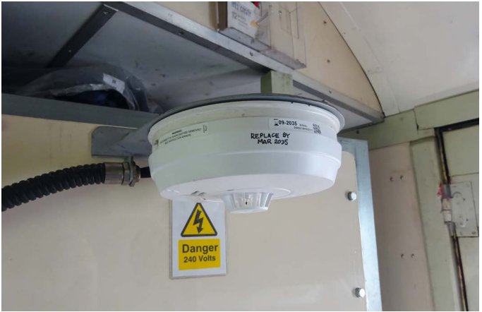
New heat alarm fitted inside Electrical Control Cabinet.
