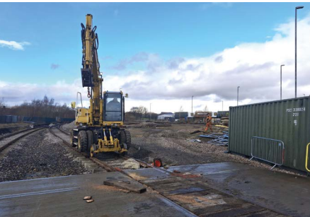
Above: Pit boards have been installed at the outside pit allowing rail traffic to run over them and allows us to maintain the pit. It also gives a rail access point (RAP) for the road rail vehicle (RRV).
