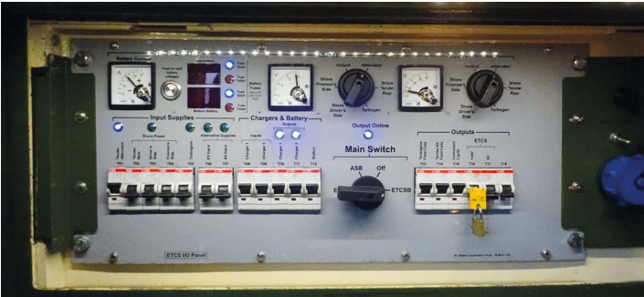
Tender ADA charging ETCS batteries at around 6A.
