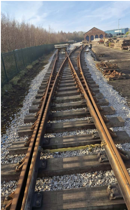
Above: Turnout Number 4 is under construction. This is the turnout from the run round loop to the south end of the 1861 shed
