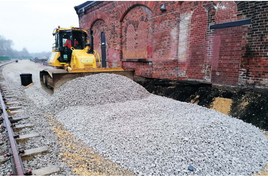
Above: In January the formation for the run round loop was finished and the ballast levelled by a GPS guided dozer before impact rolling.
