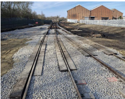
Above: The level crossing for Network Rail to gain track access with vehicles was constructed over our running line and run round loop, this is also gives us a RAP for the RRV which is essential as the run round loop must be built from the running line.
