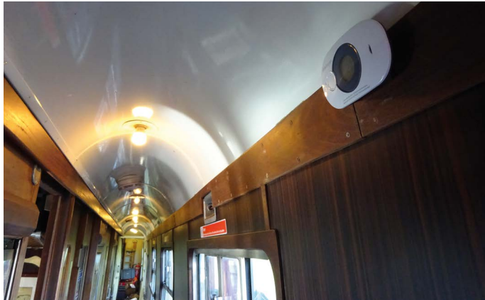
New Carbon Monoxide alarm fitted in coach corridor close to kitchen.
